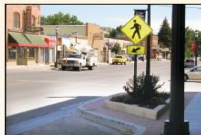
BULB-OUTS, OR EXTENSIONS of the sidewalk at either end of a crosswalk, make the distance people have to cross shorter and make it easier for drivers to see the people trying to cross the street.
