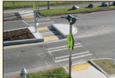
MEDIAN ISLANDS provide a safe place in the middle of the road for people to stop and wait for traffic. If there is a median island, people do not have to wait for traffic to clear in both directions. They can cross when traffic is clear in only one direction.
