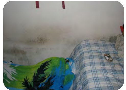
Keeping furniture and other belongings at least three inches away from walls will help prevent mold like this from growing.
