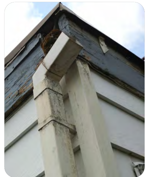
This roof has no gutter, so the downspout is clearly not serving its purpose.
