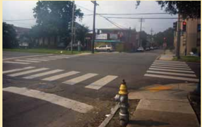
Continental crosswalks, shown here outside Drew Elementary/ARISE Academy are designed for higher visibility and longer lifespan.
